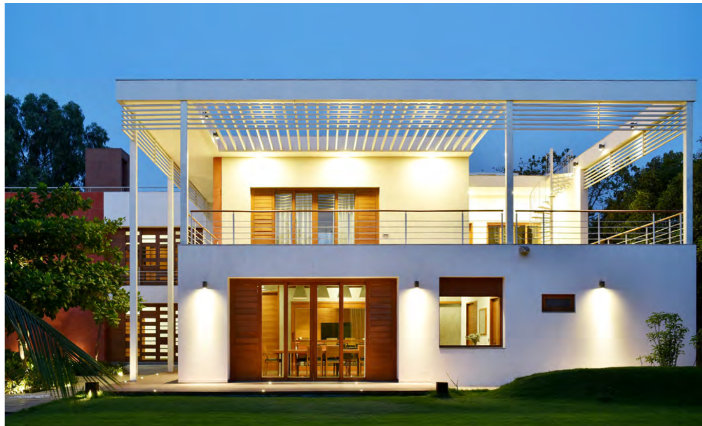
↑ The built form of the Pool House mirrors the semantics of the Pavilion – The steel columns and horizontal louvers are reproduced in the balcony and open areas to create cohesion between the old and new structures.
